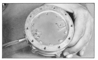
20. Insert Seal Retainer Washer (14) in slot to hold the Lip Pin Seal (9) in place.
